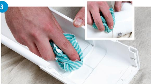
Any surplus solvent cement should be removed immediately with a damp, clean, lint free cloth. Leave sitting for 10 minutes.
