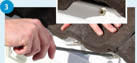
Secure spouting to fascia using a screw at the point furthest from the expansion outlet in the same run. This will control movement to and from the expansion outlet.
