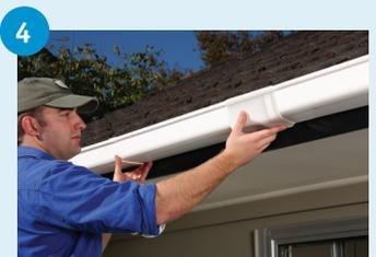
Roll the end with the expansion joiner into place by first engaging the back lip and then clicking front lip into position. Then solvent cement the joiner at the other end.
