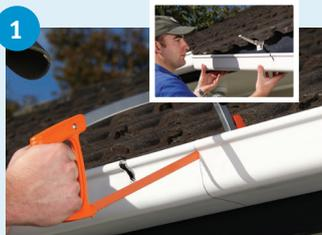
Block spouting with cloth to create dry working area. Mark and cut 50mm inside bracket either side of damaged area.
