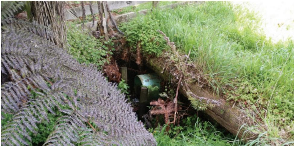
Outlet(agriduct) of lake to supply pump to fill new tank.
