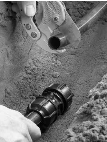
1. Cut Pipe Square Cut the pipe square. There is no need to prepare the pipe end. Chamfering or lubrication is not required.
