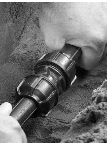
3. Pipe Insertion Insert the pipe until the stop is felt.
