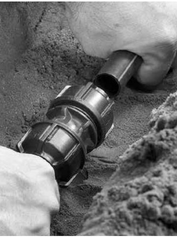
6. Disassembly To disassemble the fitting simply loosen the nut using a wrench until 2 threads are showing. Pipe will be released and can simply be pulled out of the fitting.
