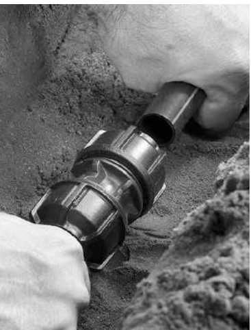
2. Ready to Use Position The fitting is pre-assembled and ready to use, however always ensure the nut is fully relaxed and 2 threads are showing before inserting the pipe.
