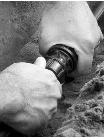
4. Nut Tightening The nut should be tightened by hand and then firmly with a wrench. Tighten the nut all the way to the flange on the body of the fitting.
