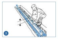
Dig a trench with adapted measures (10cm around the channels). Realise the concrete bedding according to the required depth.
