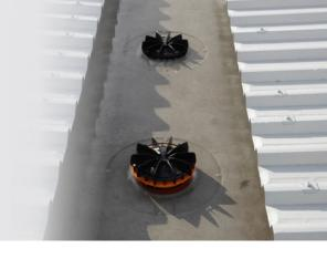
Akasison siphonic roof drainage is a concealed system that rapidly drains rainwater from commercial building roofs. The system siphons the water off roofs while maximising space due to its unique pipe system design, it uses fewer downpipes that are smaller than a conventional gravity drainage solution.
