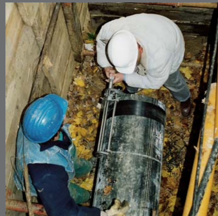
Demonstrating a scraper tool right at the construction site.
