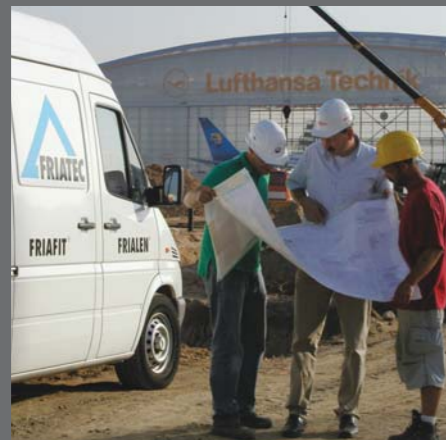
Practical based construction site training by your FRIATEC adviser.
